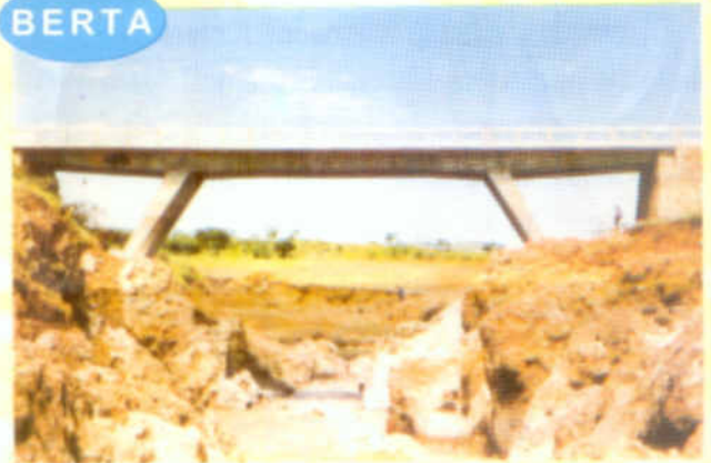
Bridge over Tekezie River - 43 mt long
